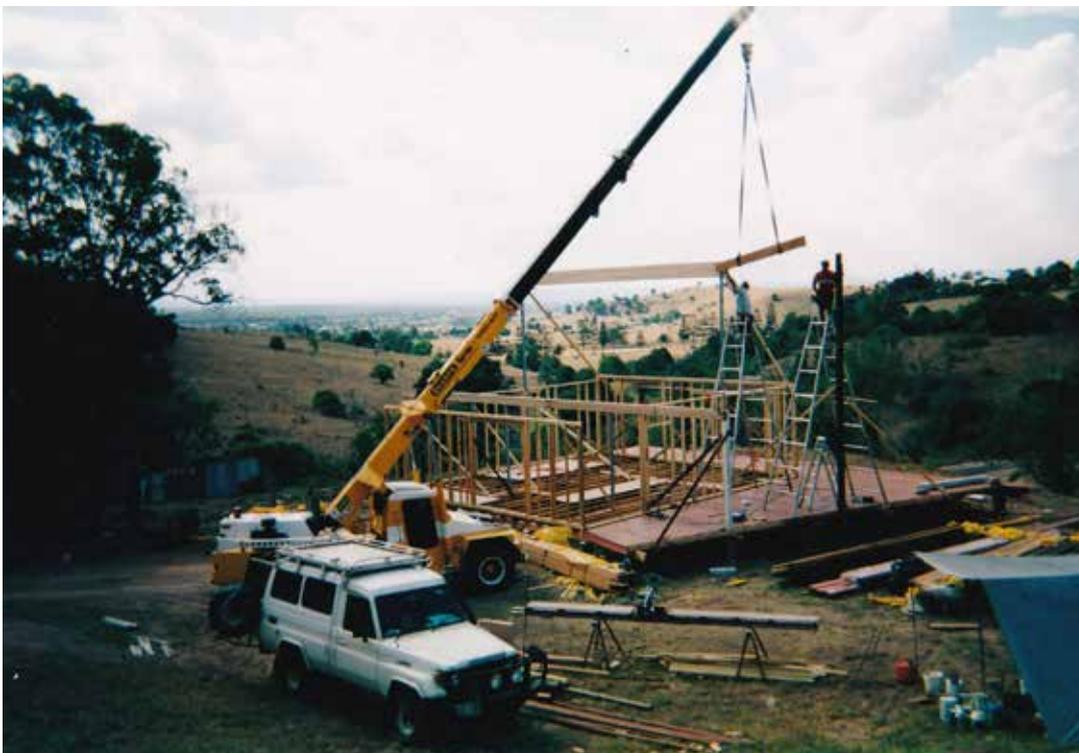
*The crane putting the ridge beam on the Western Wing of the Homestead. We lived in a shed with no hot running water at the top of our property for 18 months while we constructed the Western Wing. When we first moved into the shed Troy told me "Don't worry Kathy, we will only be in the shed for a couple of months". The big wooden chopping board in the kitchen is an off cut from the ridge beam.*
