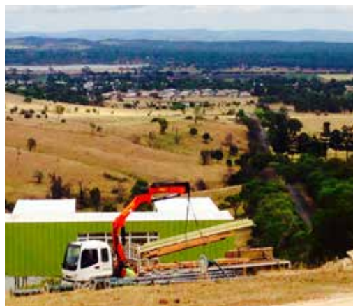
The timber arrives ready for construction.
